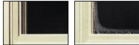
I.G. units feature Intercept "Warm-Edge" technology that reduces condensation problems around the window perimeter. Compare the Intercept insulating glass window (above left) with a conventional insulating glass window (above right). Both windows have Low-E glass and argon gas infill. The difference is the Intercept Warm-Edge Spacer.
