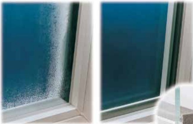
Traditional Metal Spacer The metal edges conduct cold from the outside, which can lead to condensation problems at the window edge.
